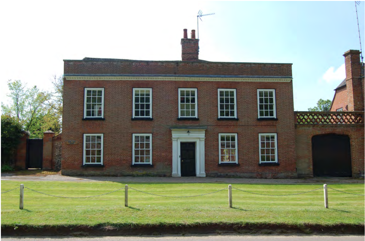
Picture 1.13 Home Farm House, originally dating from the 17th century it was refaced with brick in the 18th century.
