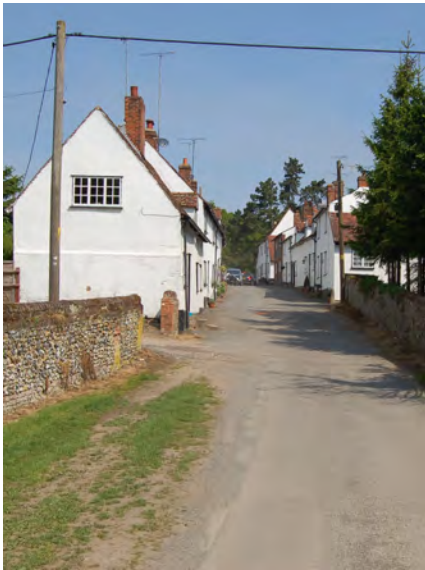
Picture 1.18 Overhead services on utility poles are somewhat disruptive in the streetscene.
