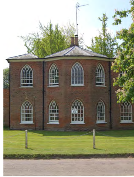
Picture 1.4 Elegant 'Gothick' 2-centred arched form windows are employed to dramatic effect on Lion House.
