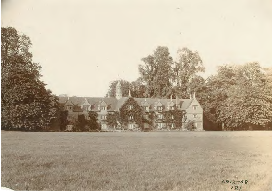
Picture 1.24 The stable block probably around the end of the 19th century from an image donated to Saffron Walden Museum in 1912. (Reproduced courtesy of Saffron Walden Museum).
