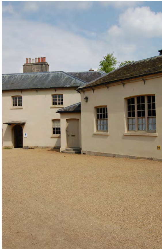
Picture 1.23 The range of 18th century colour washed service buildings extending to the north and west of the main house.
