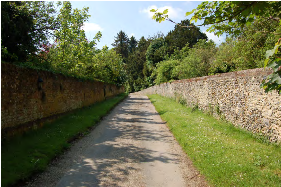
Picture 1.16 A fine run of flint walling with semi-circular brick caps lines the long approach to St Mark's.
